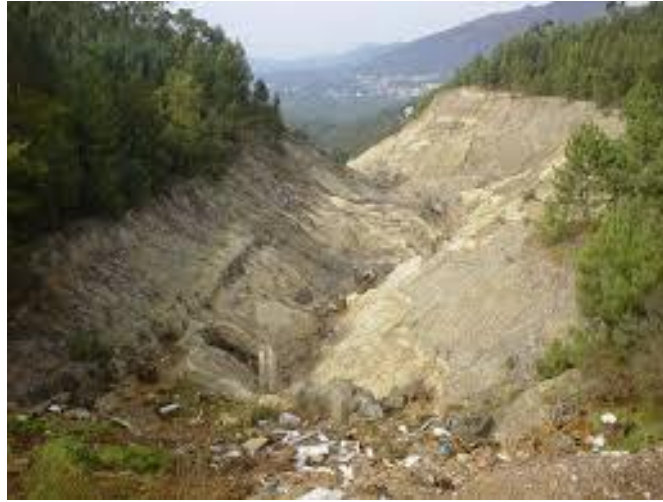
Figure 6. Terramonte mining waste led to the collapse of the heap and the materials started being transported along the Ribeiro da Castanheira to the Douro River.
